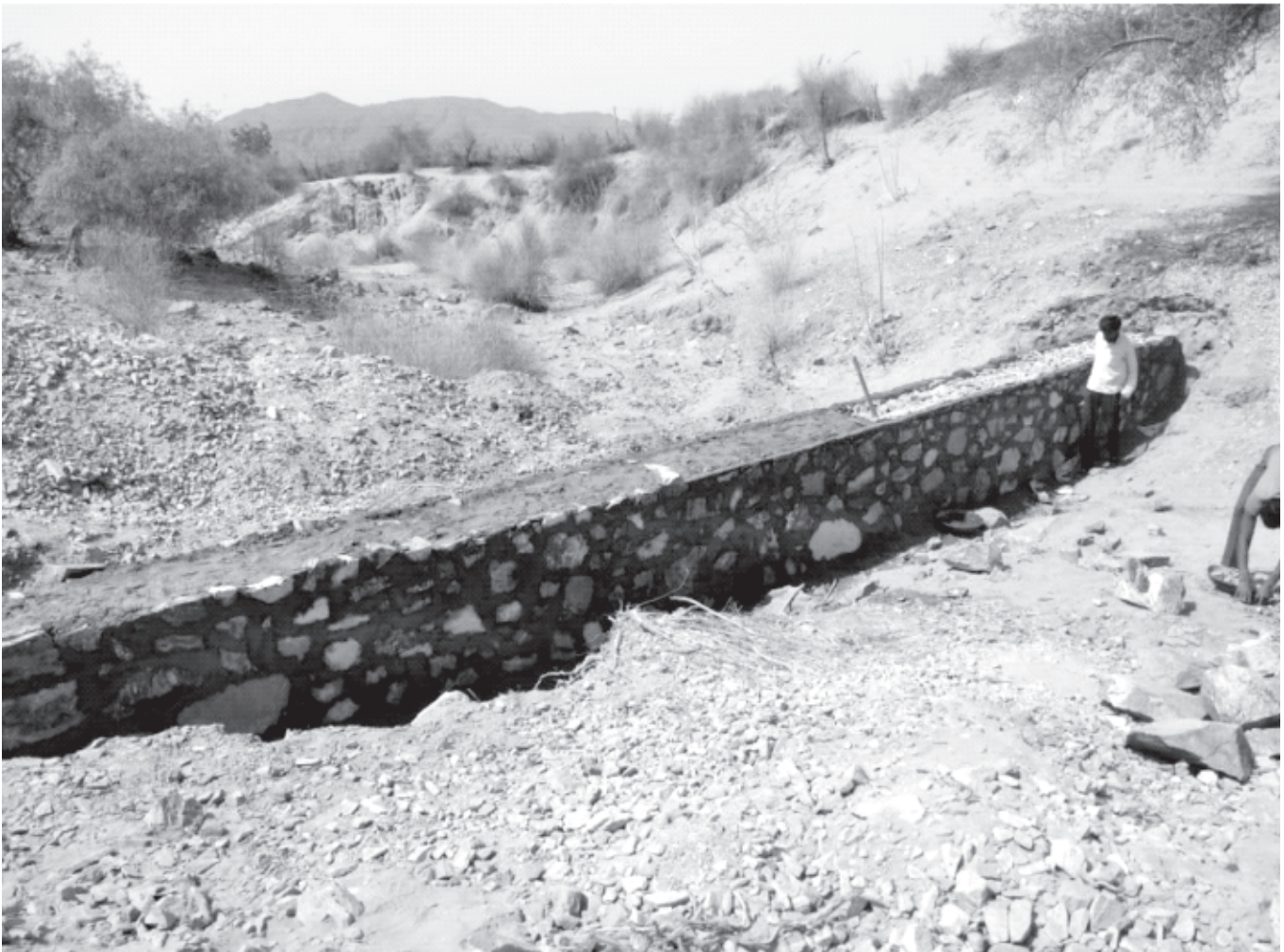
Construction of masonry check dam in progress
