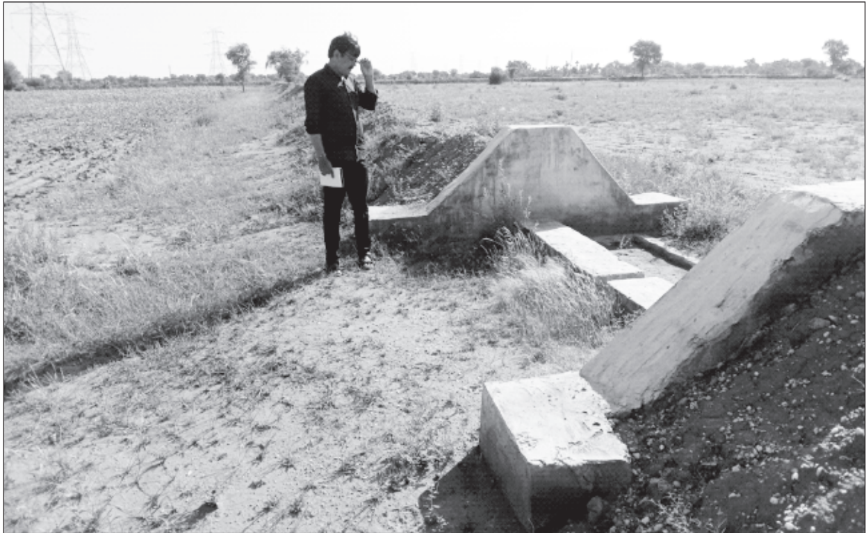
A newly constructed khadin as part of the WNHT project
