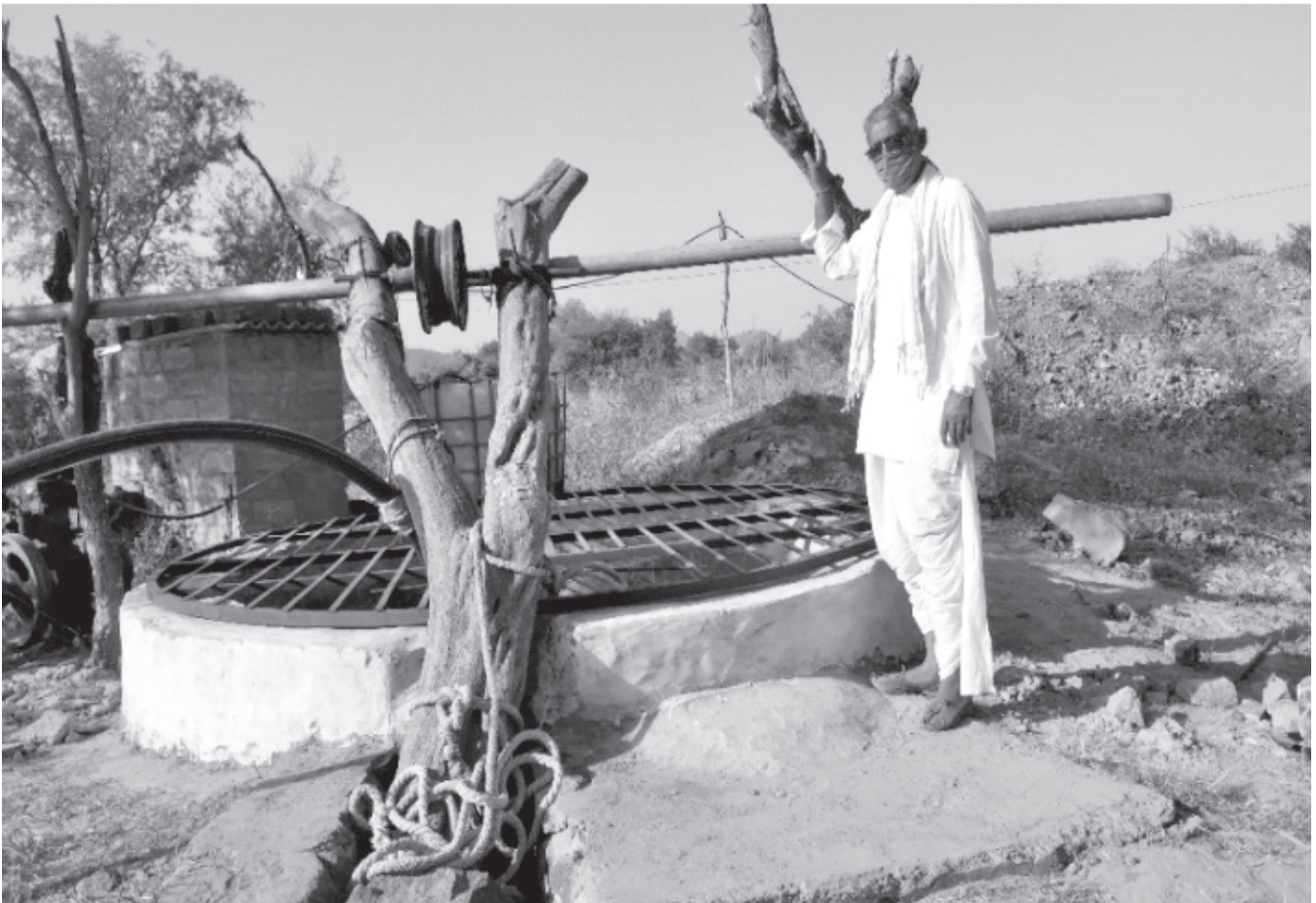
A renovated beri as part of the WNHT project
