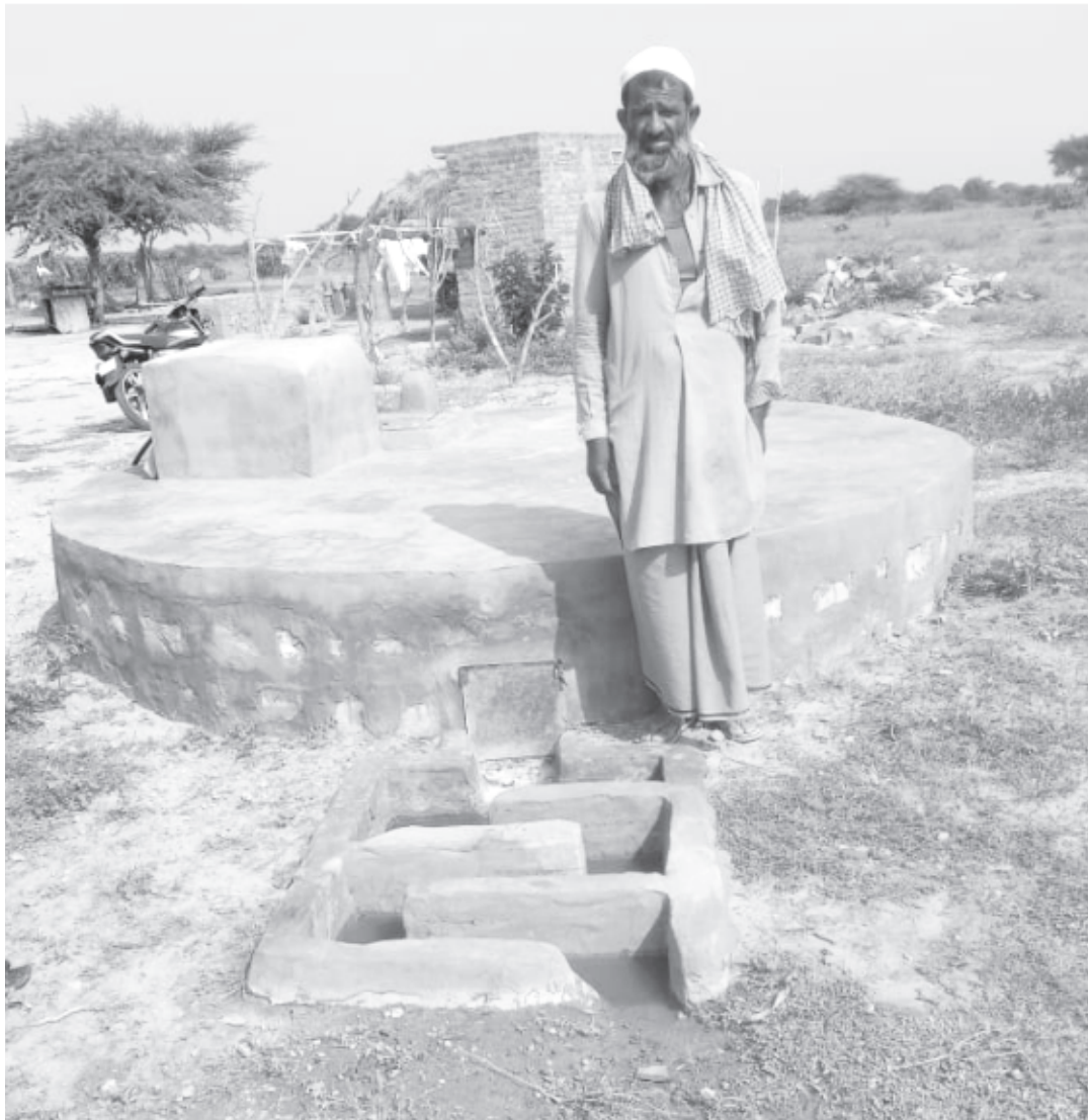
Kasim with his newly built taanka in Bohranada village, Jodhpur district of the Thar
