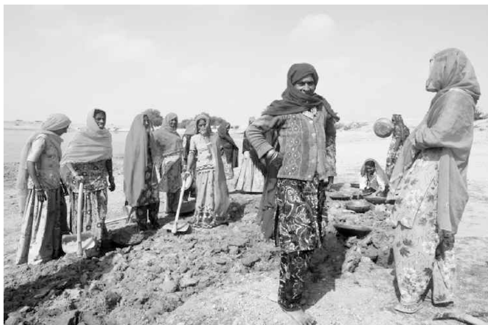
Women working at a pond renovation site
