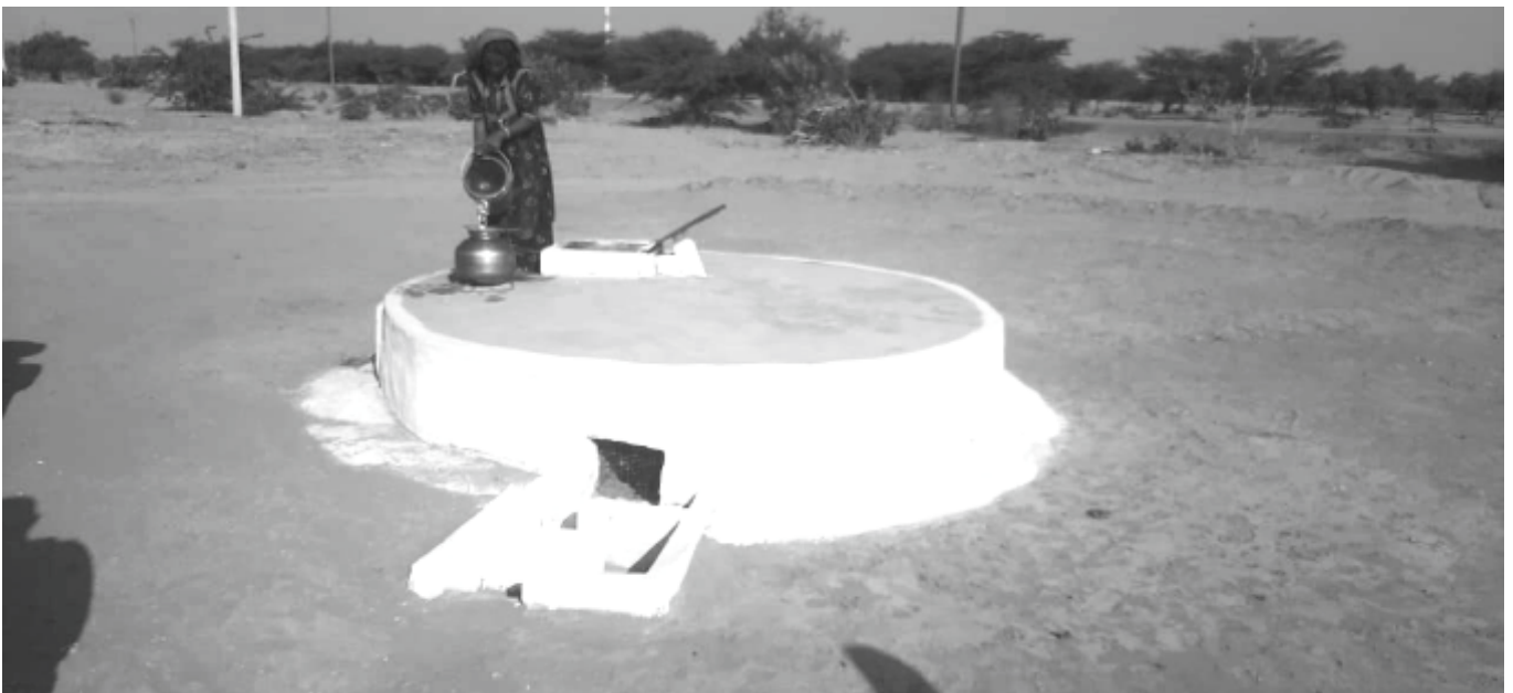
A taanka with silt trap constructed under the project and the beneficiary family
