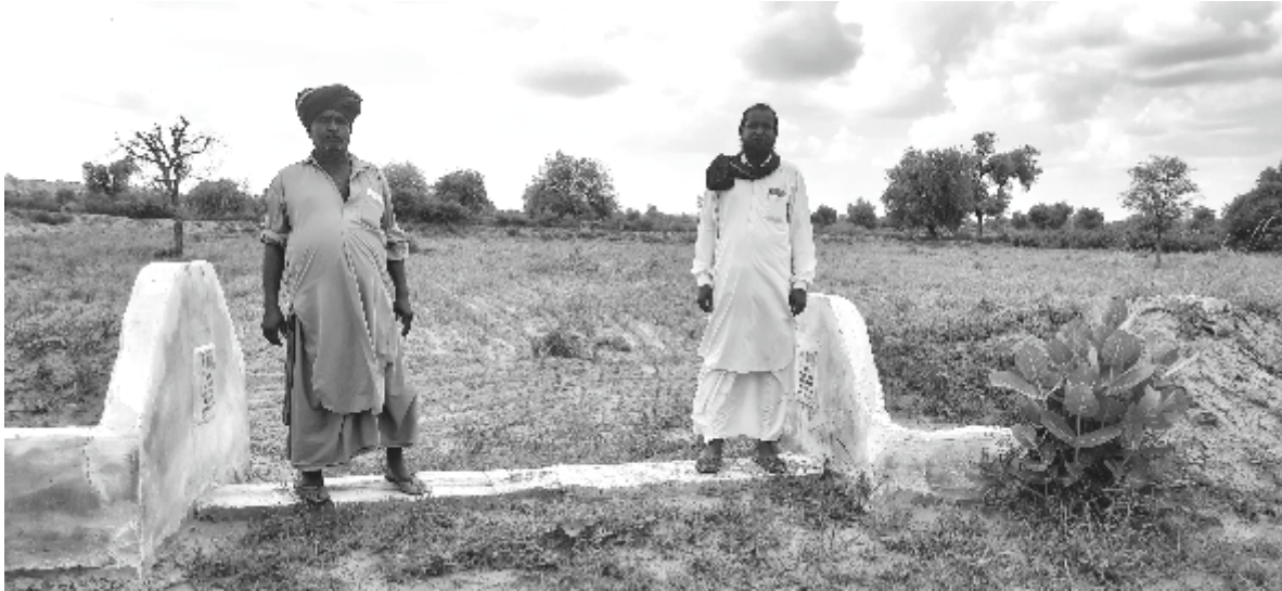
Masonry spillway of khadin
