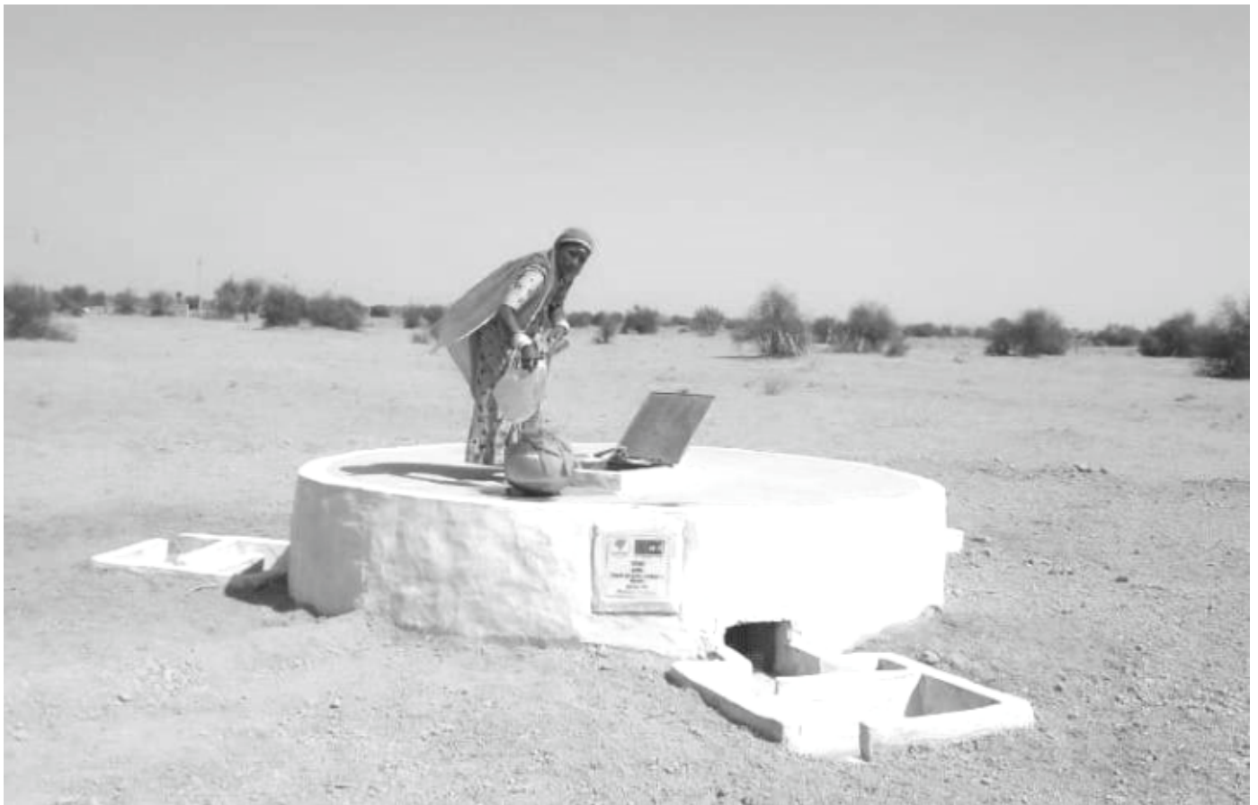
A taanka constructed by the project
