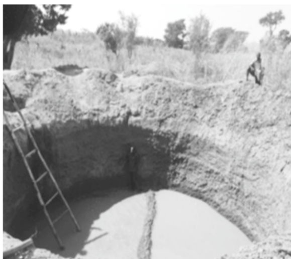
Seepage well dug by the community
