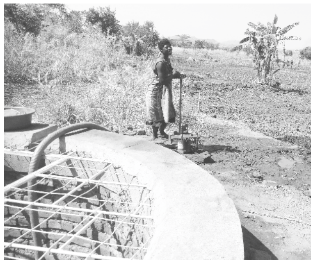
Seepage well after the masonry work—ready to store rain water
