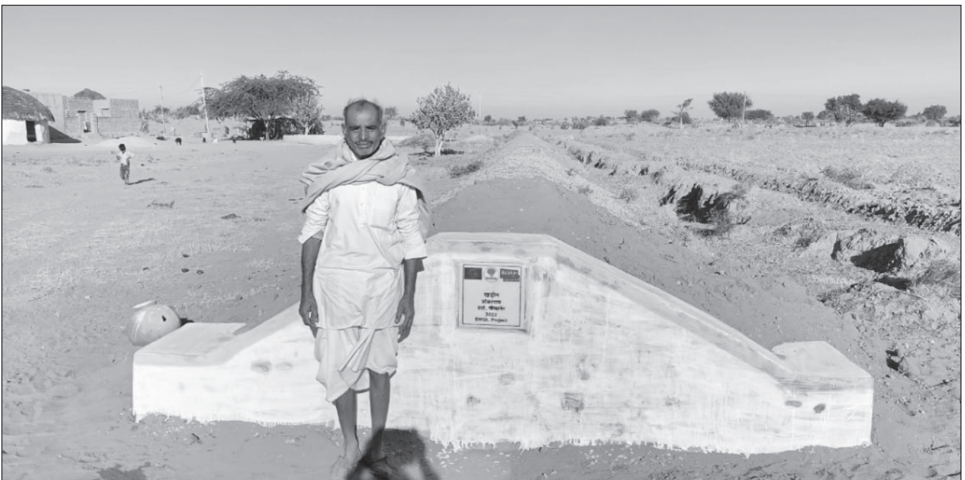
Khadin constructed at Shankar Ram's farm in Handi Village
