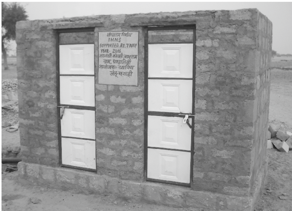
Low Water Use Toilets
